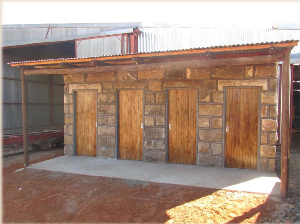
The toilet block situated at the end of the coach accommodation.
